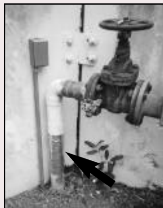
The coil is wrapped around a water pipe and protected from dirt, disturbance and moisture with weatherproof tape.
